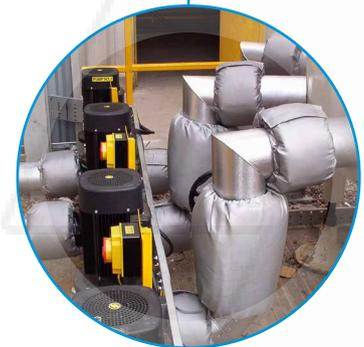
**Example 4" valve in a plant room with 50mm insulation jacket:**
