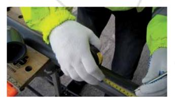
**7b.** Generally containment pipe needs to be shorter than the carrier pipe. This distance can be worked out from the data on pages 90-91. A2 - A1 = Additional length of carrier pipe eg. for  $^{1}/^{2}$ " # 2" (90° Elbow) this equates to 35.1 - 12.7 = 22.4mm
