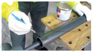
**6.** Without delay assemble the outer joint as described in step 4. This process (points 3-6), can be repeated using standard PVC sockets to extend the pipe lengths, until there is a change of direction needed.
