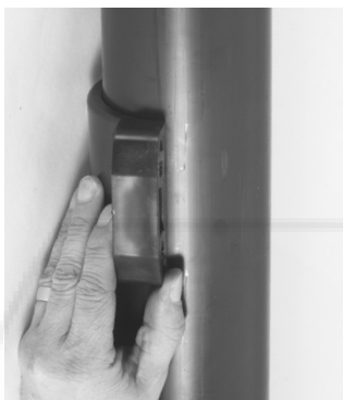
1. Position lower half of saddle around pipe.
